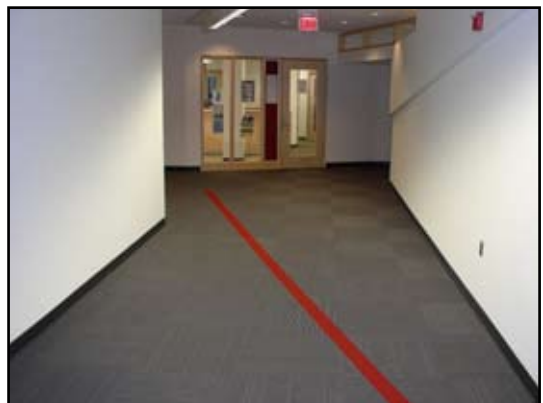
Second Floor Renovations
